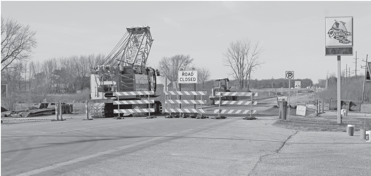
On March 21, the project was underway.
