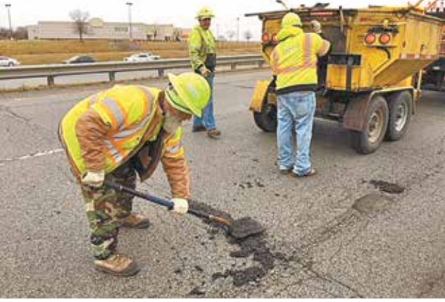
Indiana Department of Transportation crews are working to fill potholes.
